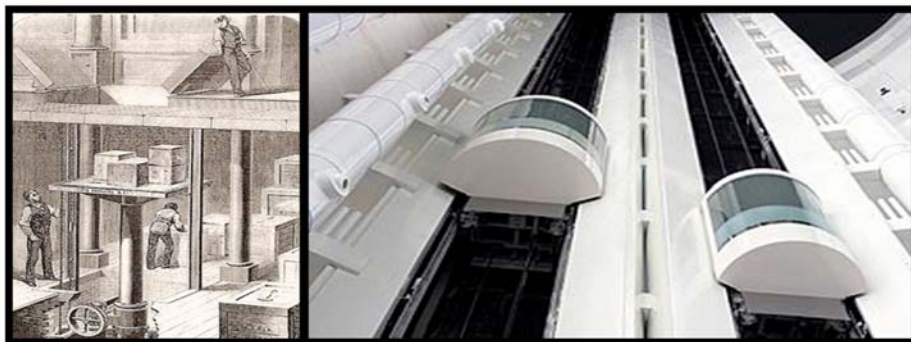
Figure 1.2: An old and a new kind of elevators
